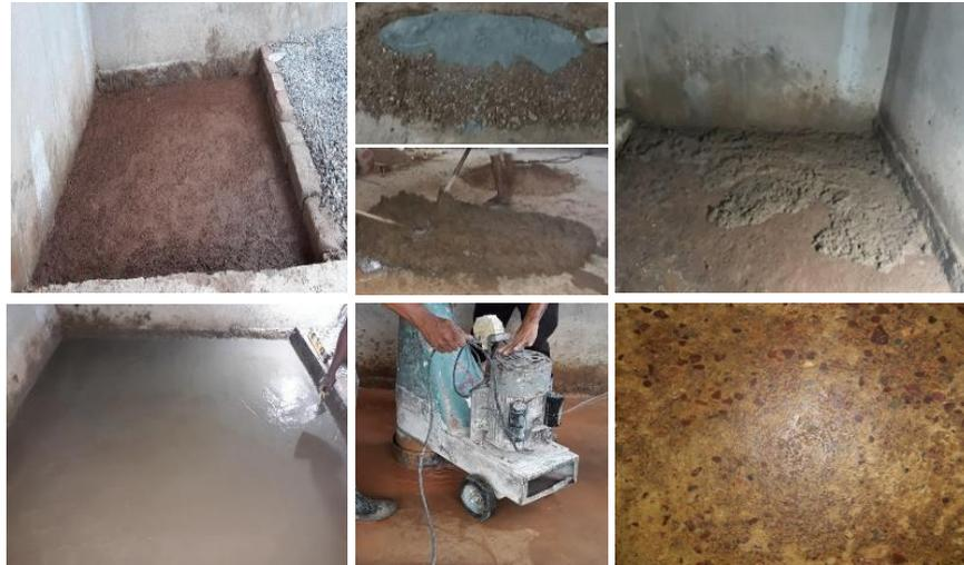
Figure1: Steps of soil floor construction
